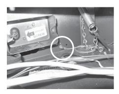
21) Connect one end of the supplied green ground wire to the lug with the nut and washer from the kit.
